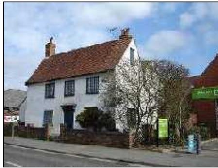
Groves House and neighbouring supermarket, London Road
