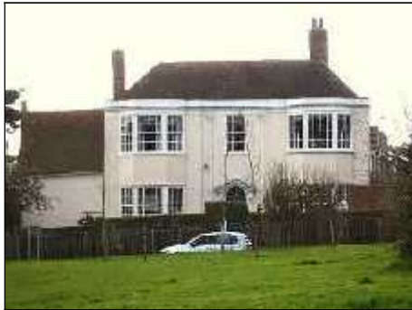
123 Sheering Mill Lane
