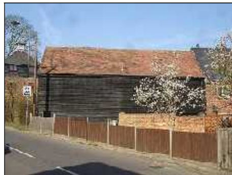
Mill Store, Mill Lane from Station Road
