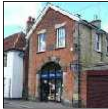
5 Church Street (the old fire station)
