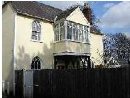
136 Sheering Mill Lane
