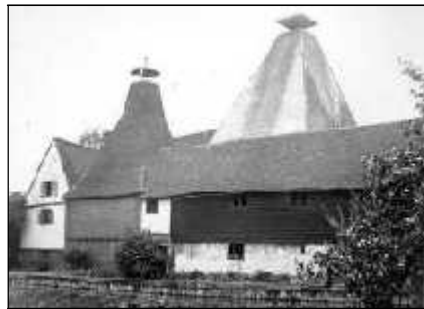
The Maltings at Sheering Mill, Station Road (HALS Photographic Collection)
