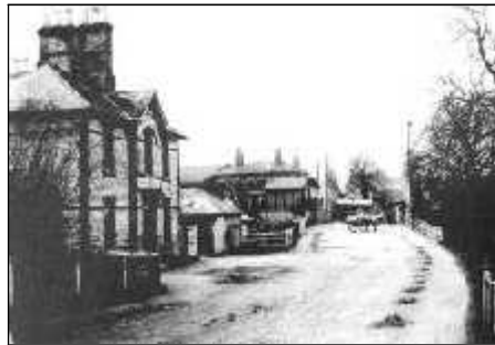
Station Road c1890 looking west. The Railway Hotel is on the left (HALS Photographic Collection)
