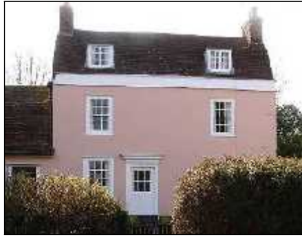
Orchard Cottage, 100 Station Road
